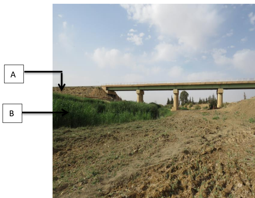
Figure 4 : La station Bedirate (2022).
