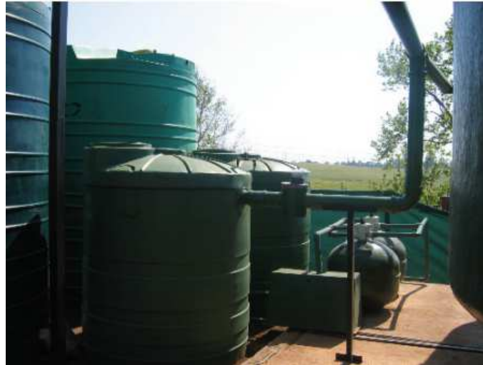
Figure I.10: Typical submerged media reactor.
