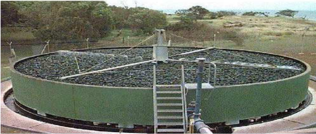
Figure I.8: Trickling filter (Wikipedia contributors, n.d.).
