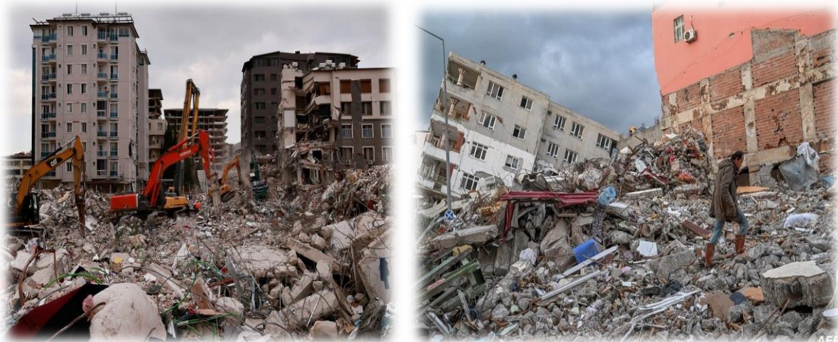
Figure 0:4. Photos from Turkey and Syria's recent earthquake [9] [10].
