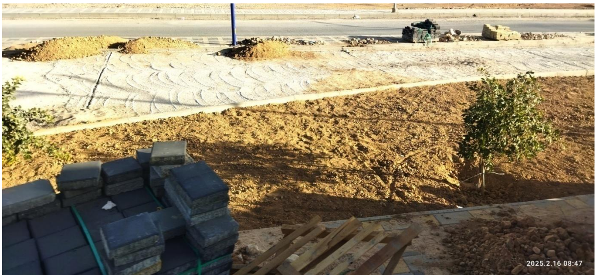
FIGURE 28 Application de la couche de ciment
