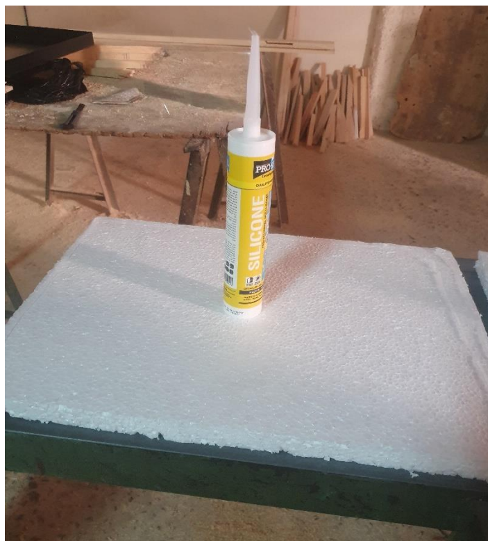
Figure III.6: fixation du polystyrène
