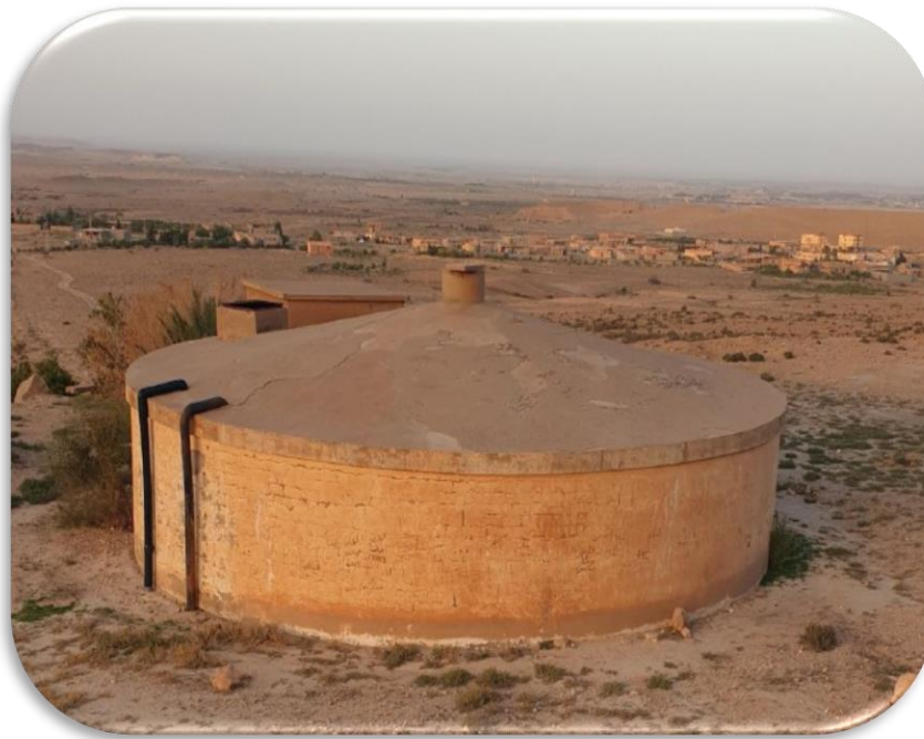
Figure II.7 Water tanks of 5000 \text{ m}^3 in Ouled sidi Ibrahim
