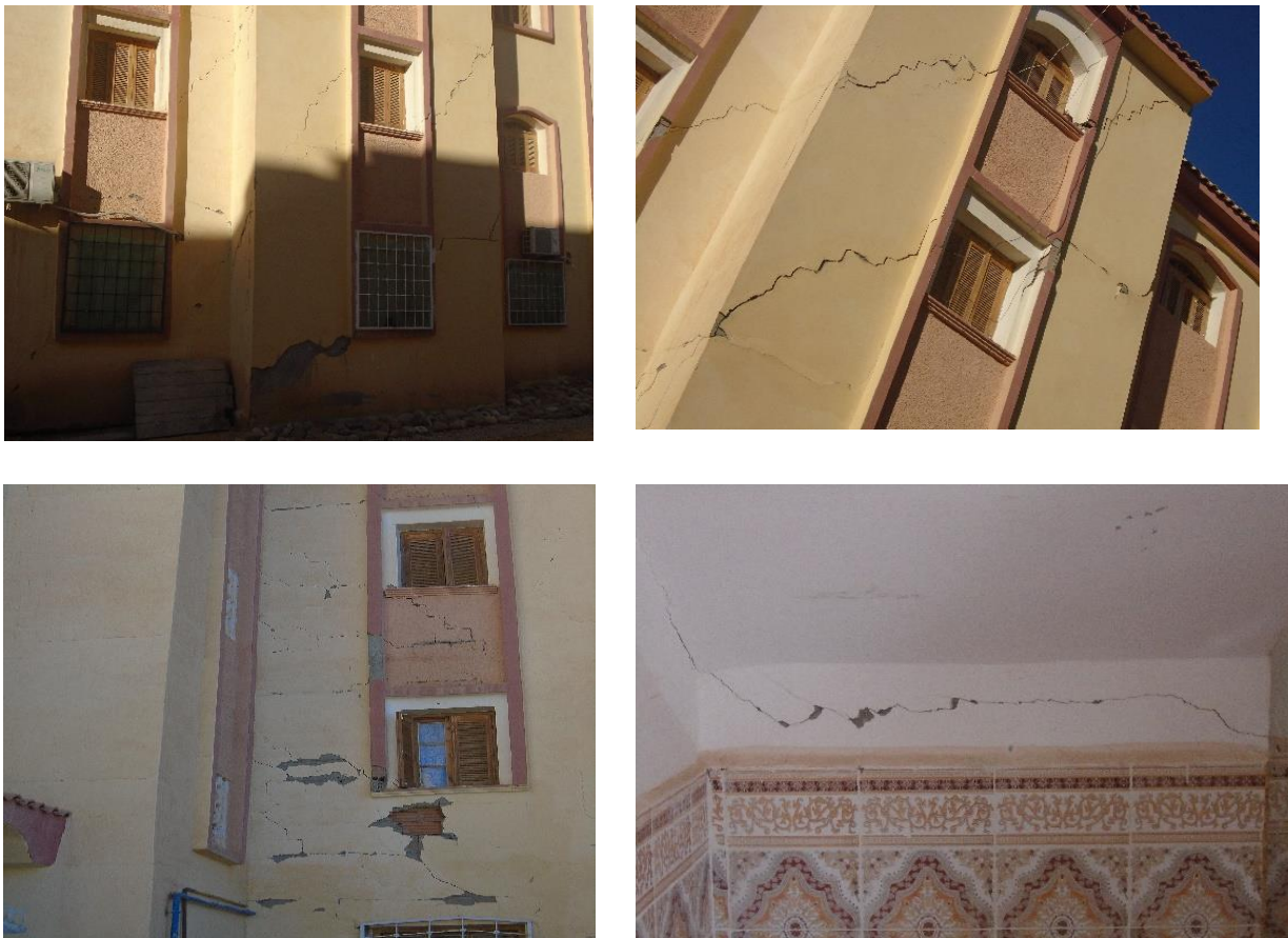
Figure III.6 Cas pathologique sol argile sablo-gypseuse (150 Logts Msila 2017)
