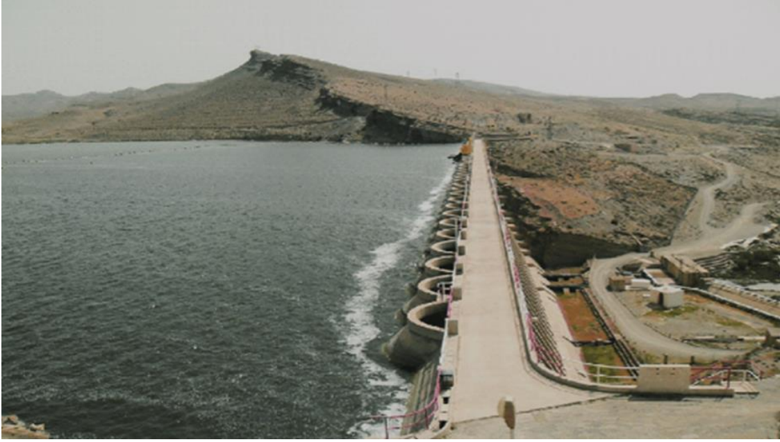
Figure I.3: Le barrage de K'sob [38].
