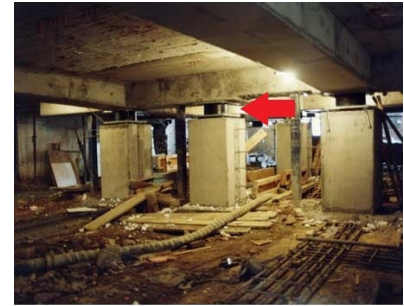
Strengthened foundation with base isolators inserted
