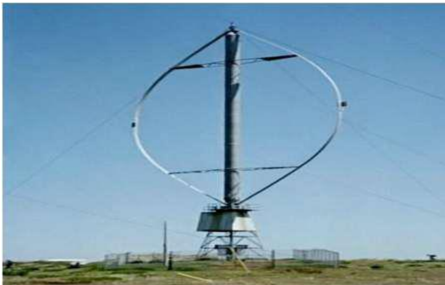
Figure (1-3): Eolienne de Darrieus
