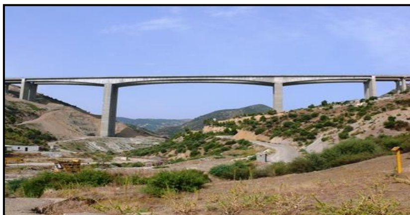
Figure 6 : Le Viaduc d'Oued Rekham -Bouira-
