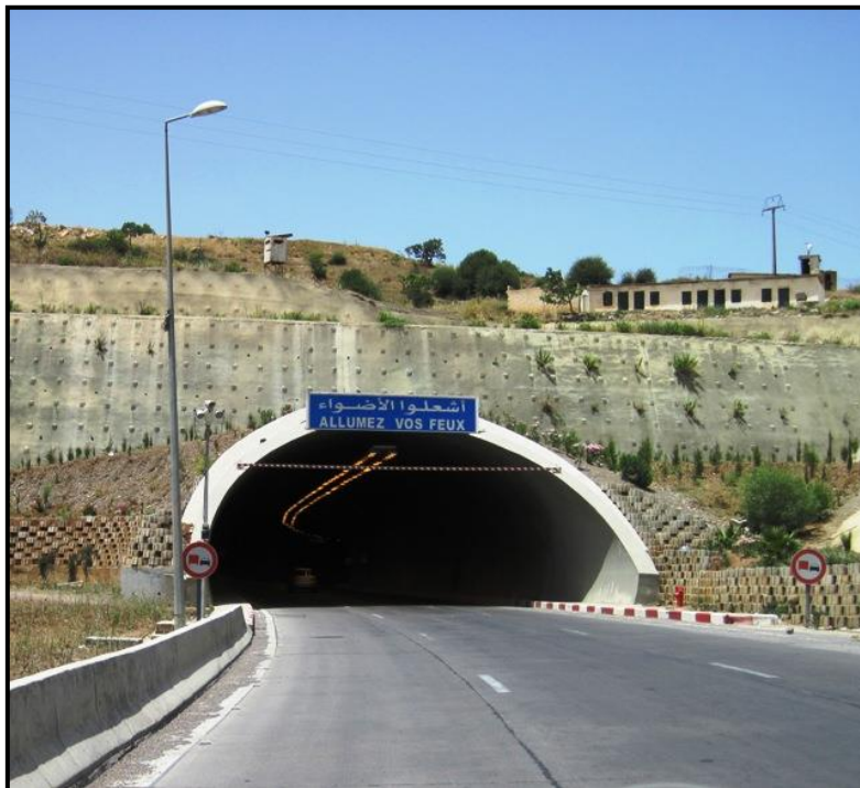
Figure 3 : Le tunnel de Djebahia -Bouira-.
