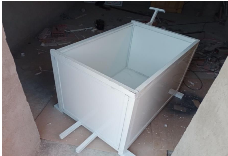
Figure3.5: Installation des panneaux sandwich
