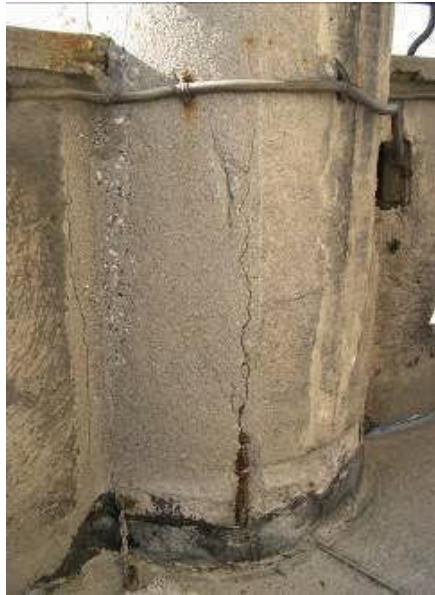
Figure 2.13 : Fissuration [21].
