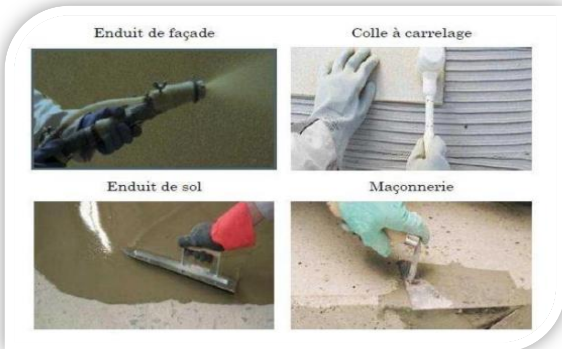
Fig.I.6 Application des mortiers [21]
