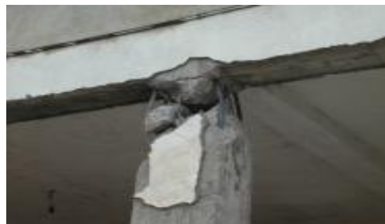
Figure II.4 : Dislocation de la section [5].
