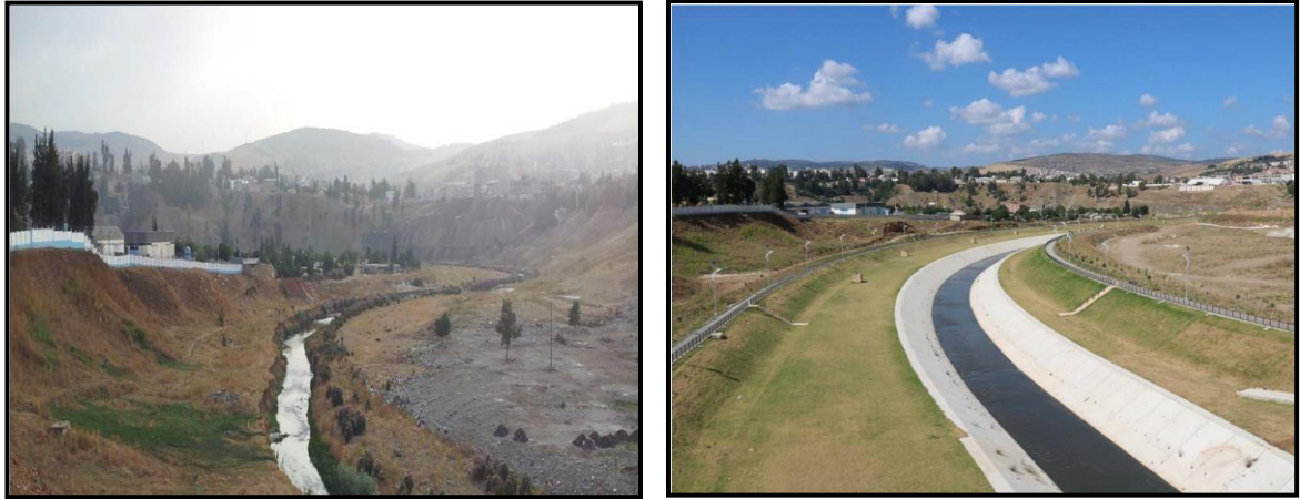
Photo n° 14: Recalibrage d'Oued Boumerzoug (Source: MRE,2018)
