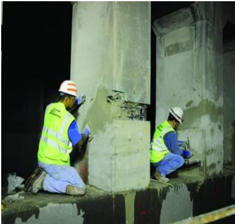
Fig.I.9. Rehabilitation project for the Lokern Road Bridge in California, USA [44].
