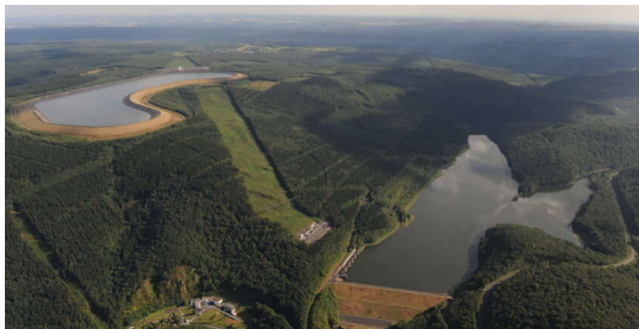
Fig II.2. The pumping energy transfer station (PETS), a proven solution for mass storage.
