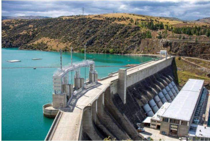
Fig.I.6. Hydraulic power station
