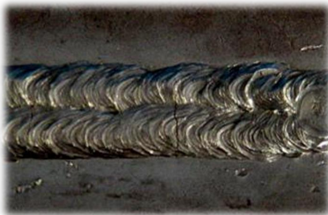
Figure (II.2) Les fissures transversales.
