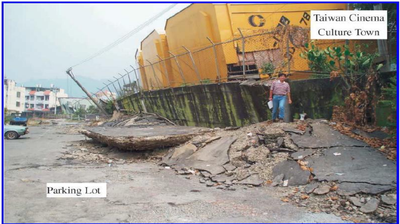
Figure 2.2 Sliding and overturning of retaining wall at site 3. [21].
