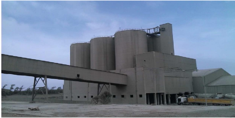
Figure I.15: Silos de stockage de ciment
