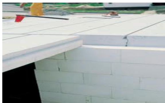
Figure V-6: Plancher en Siporex.
