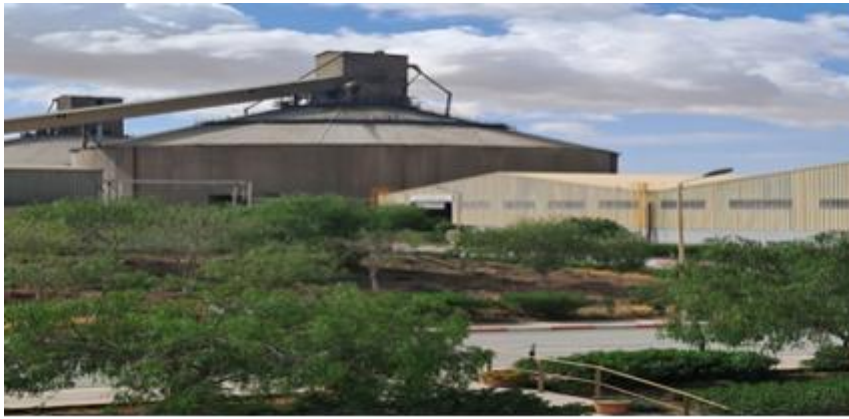
FIGURE II. 7: HALL DE CEMENT PETROLIER ET SILO CLINKER LCM
