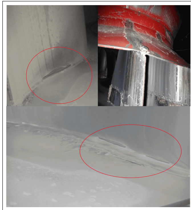
Figure 5.22: In-service erosion inspection of the Blade pressure side .
