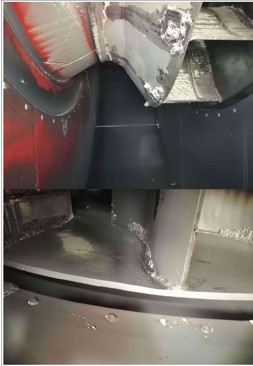
Figure 1.3: Sacrificial plates welded on the blade pressure side
