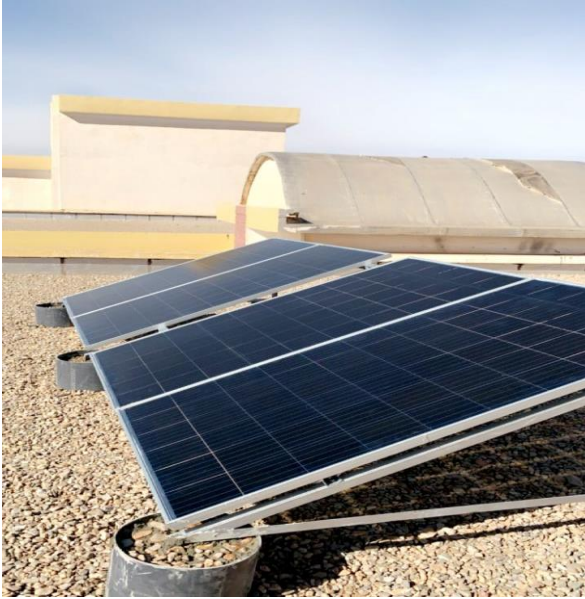
Figure III.6: Installing the Panels
