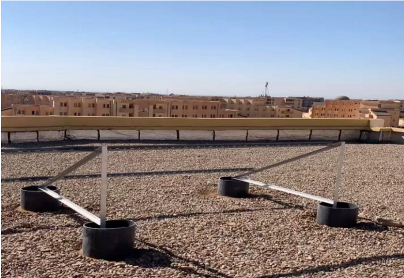
Figure III. 4: The load-bearing structure of the panels
