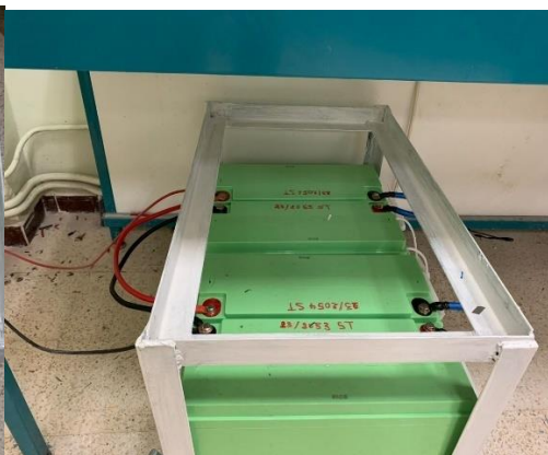
Figure III.8: Connecting the batteries
