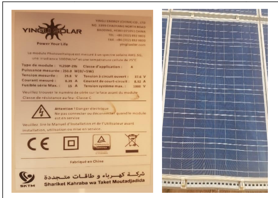
Figure II.8. The technical sheet of the PV panel and the PV module.
