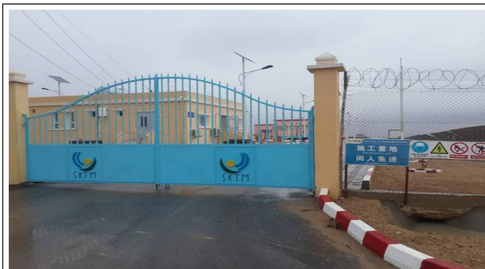
Figure II.2. Aïn El-Melh solar photovoltaic power plant
