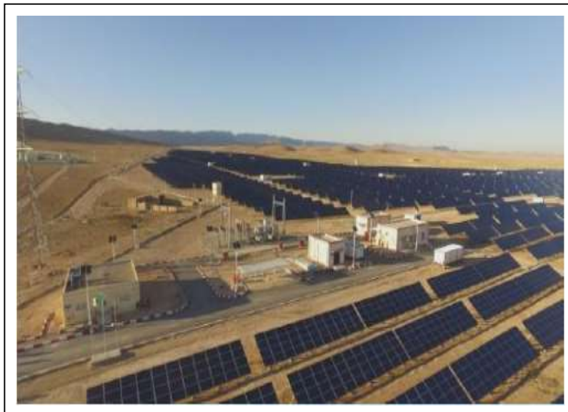
Figure III.1. 20 MWp grid-connected ground-mounted PV plant system at Ain El-Melh.
