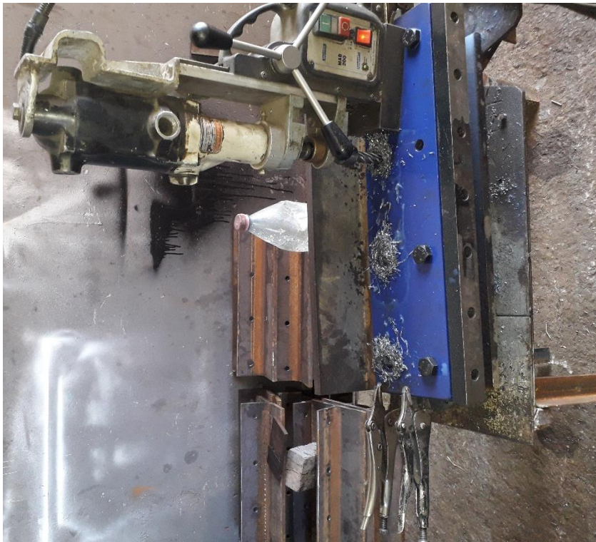
Picture C3: Drilling of the T-shape steel section
