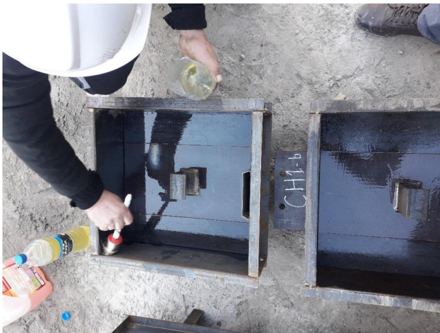
Picture C4: Elimination of steel-concrete adhesion by oiling.
