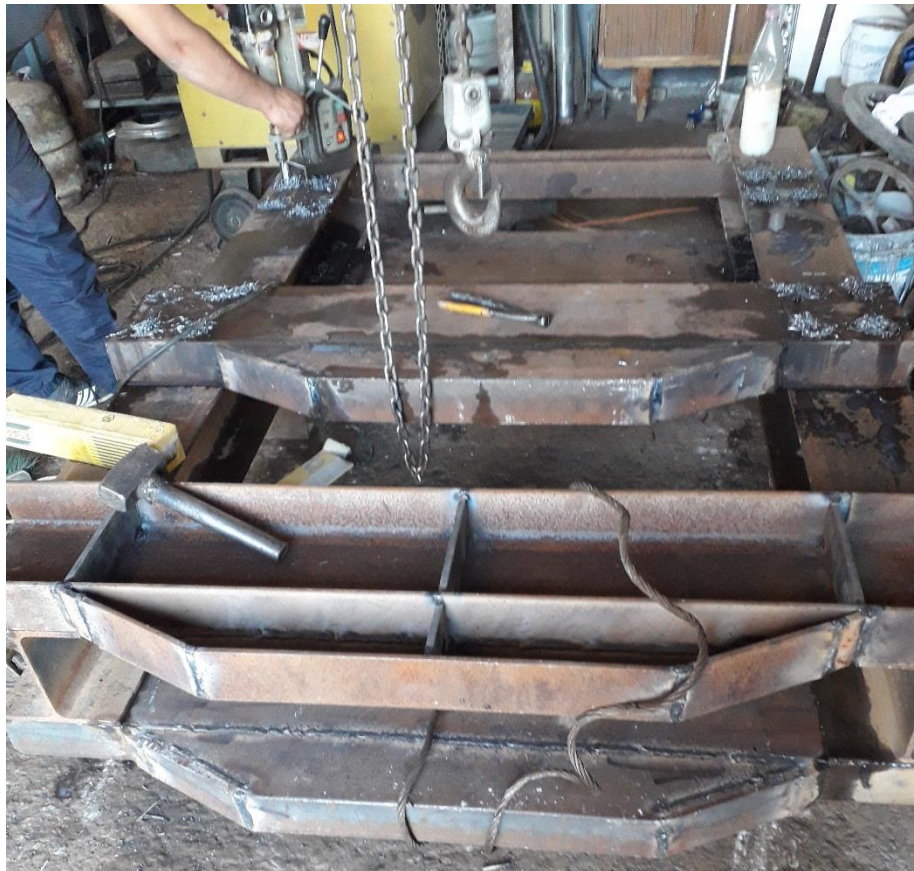
Picture C2: Drilling in the hydraulic press column.
