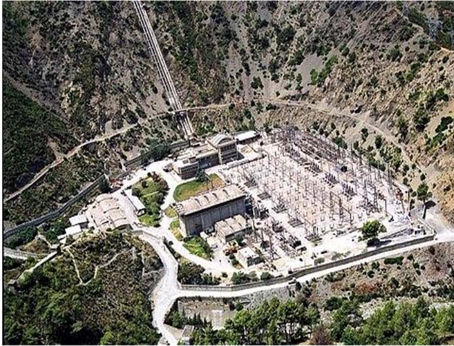
Figure 4.1: site centrale DARGUNA. [26]
