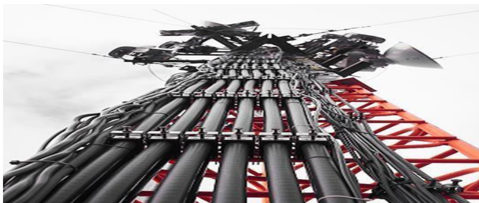
Figure I.9: câbles coaxiaux (Feeder)
