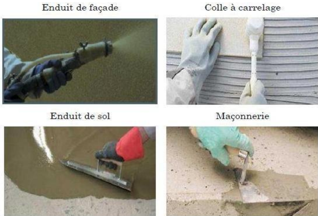
Figure (II.1) : Application des mortiers [18].
