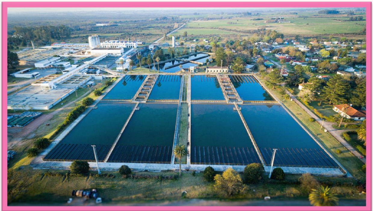
Figure 2: Station d'épuration (STEP).
