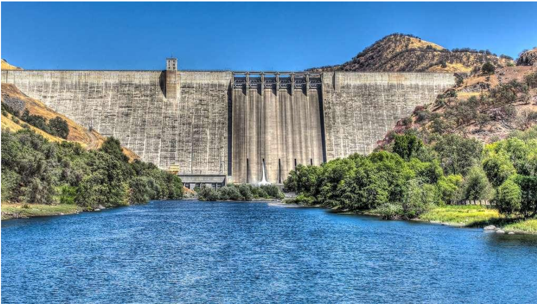
Figure II.6: Le barrage-poids de Pine Flat
