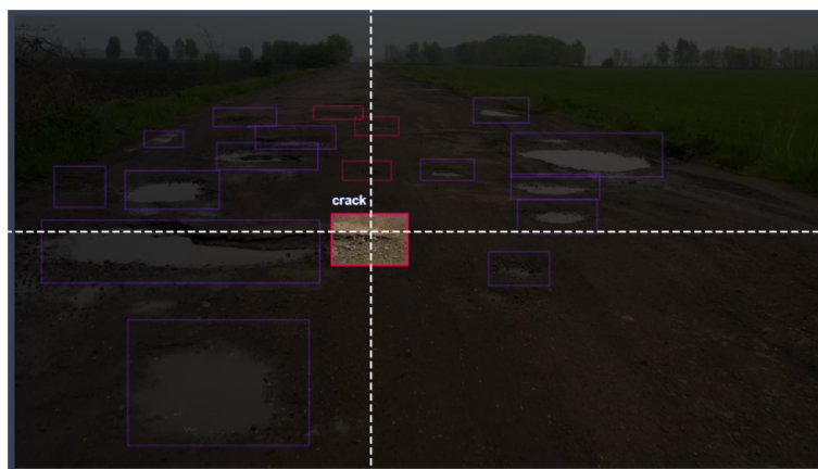
Figure 3.17: The annotation process on crack
