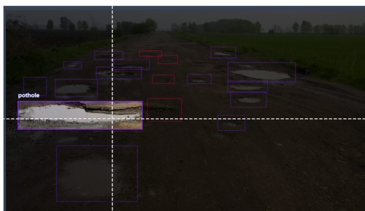
Figure 3.18: The annotation process on pothole
