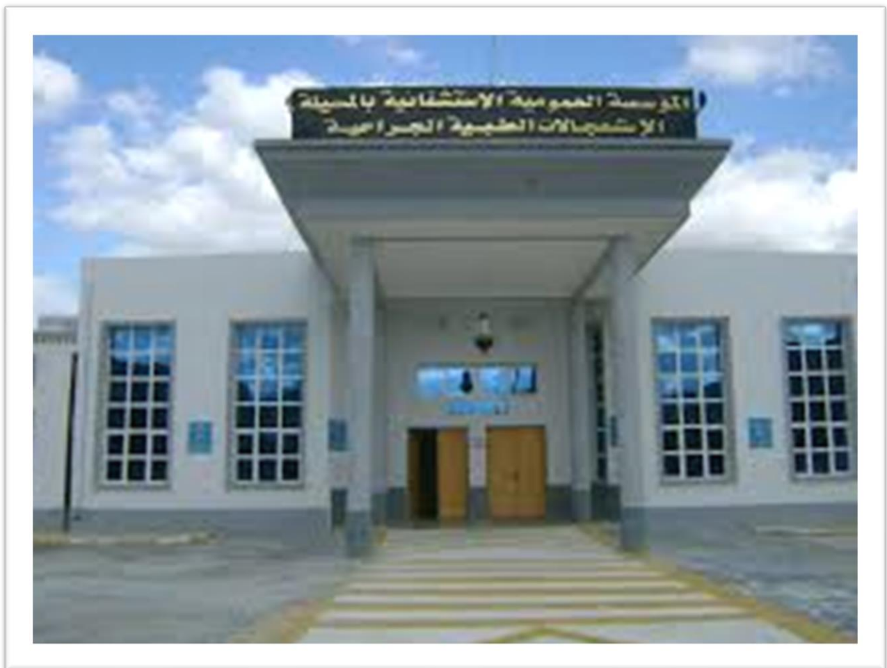
Figure 1 :Al Zahraoui Hospital entrance
