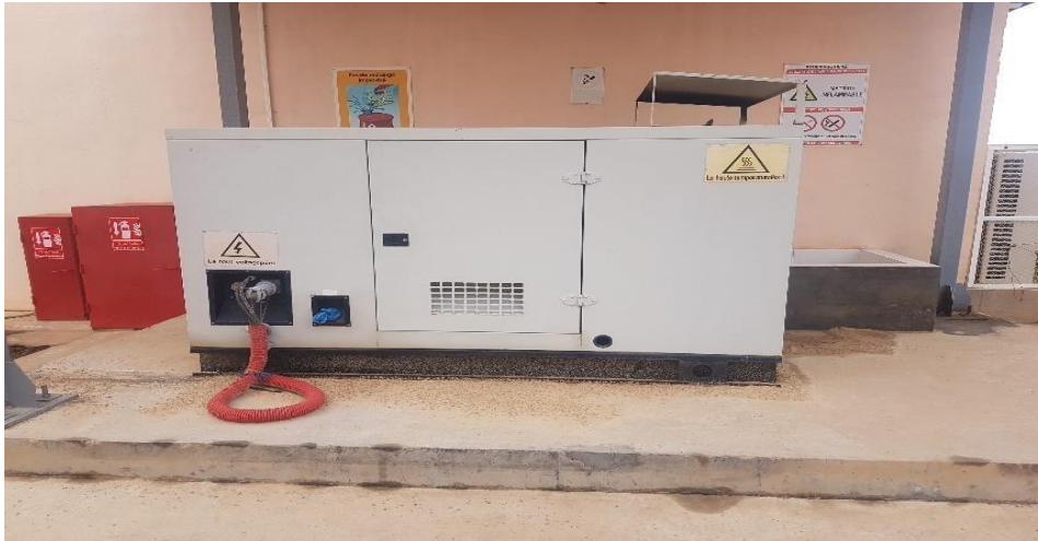
Figure II.12. Diesel Generator.
