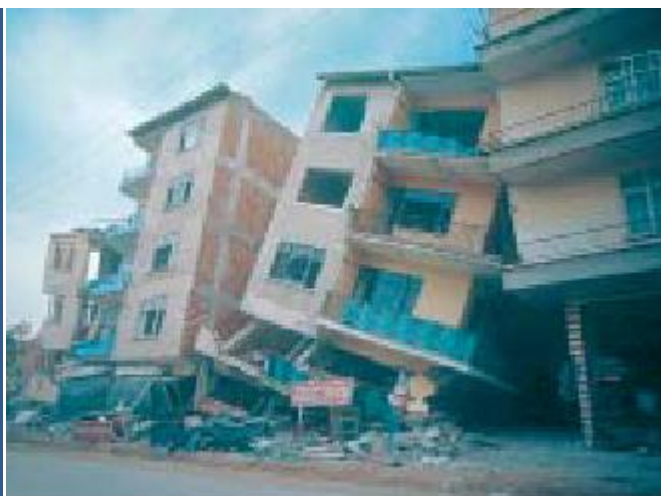
Figure III.19 : Etage souple[34]
