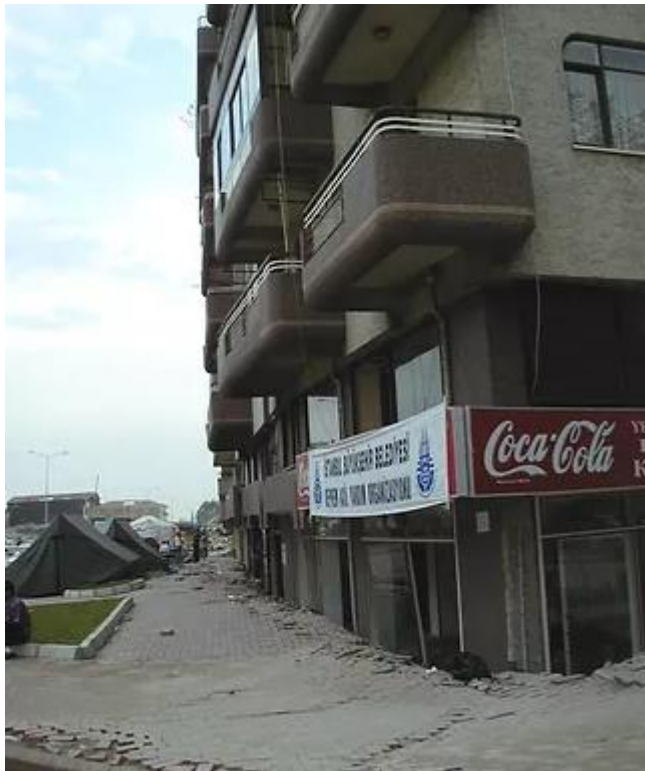
Figure III.23 : La liquéfaction (Turquie 1999).
