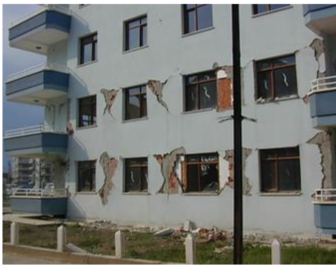
Figure III.17: Fissures en croix.
