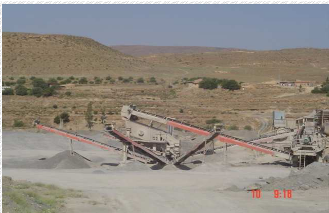
Fig.4 Station de concassage 100T/H
