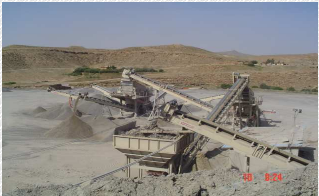
Fig.5 Station de concassage 170T/H
