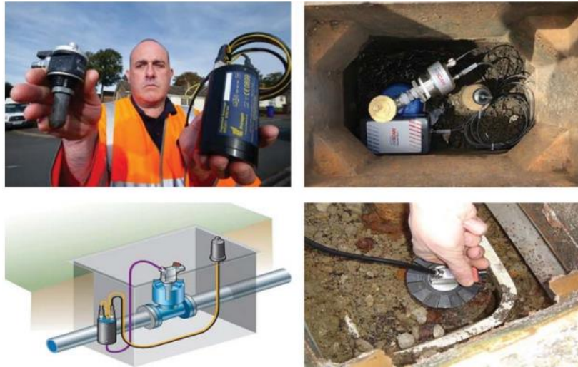
Figure.2.16 Example of hydrophone installation. [14]
