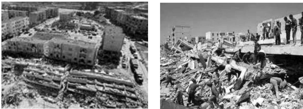
Figure I.10. RC buildings damaged by recent earthquakes Ain Temouchenet 1999 and Boumerdes 2003. [15]
