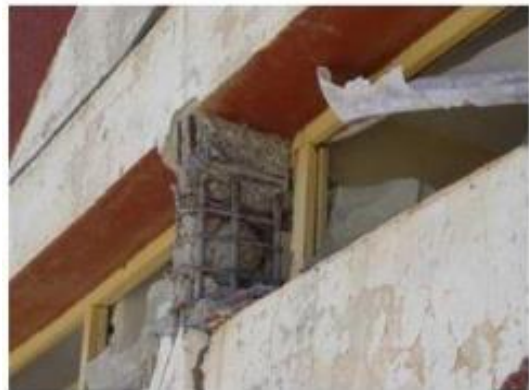
Figure III.4 : cisaillement d'un poteau Court [41]
