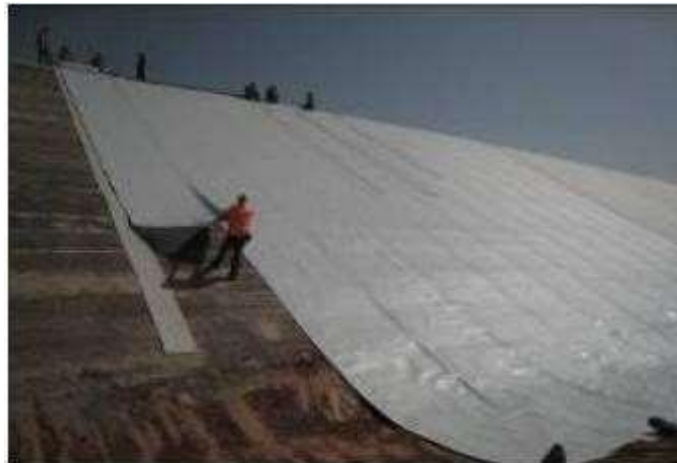
Figure 1.8: Pose de géomembrane (Barrage de Sar Cheshmeh, Iran)
