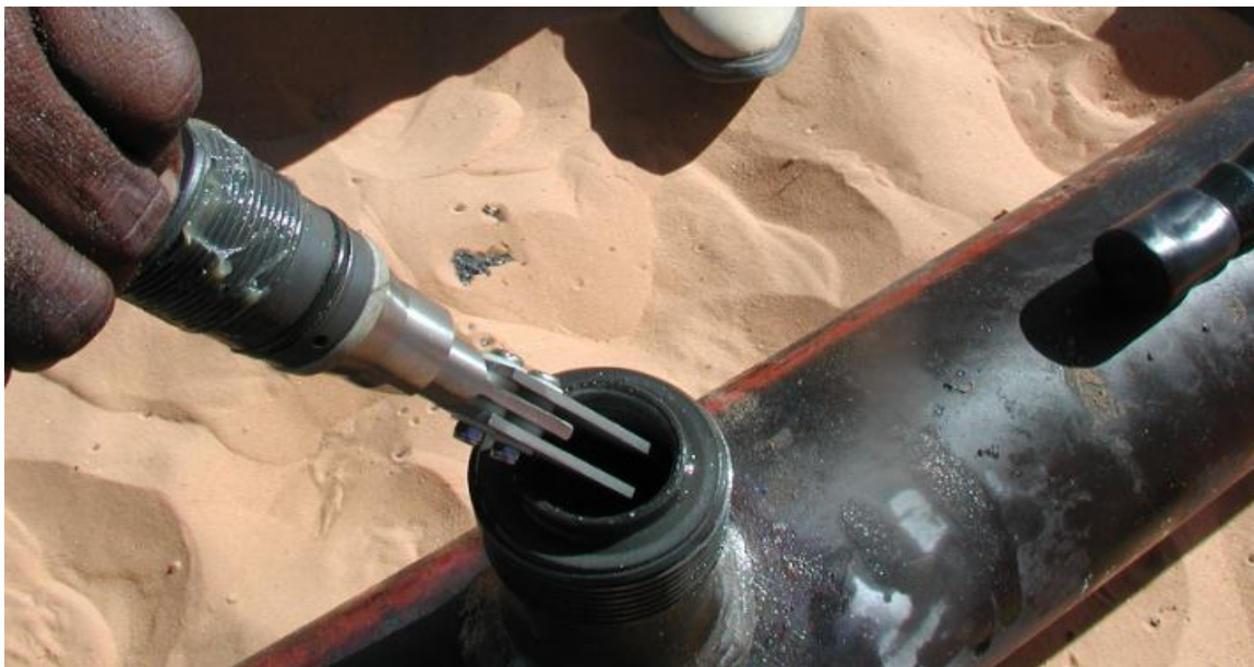
Figure(4.13): placement coupon.
