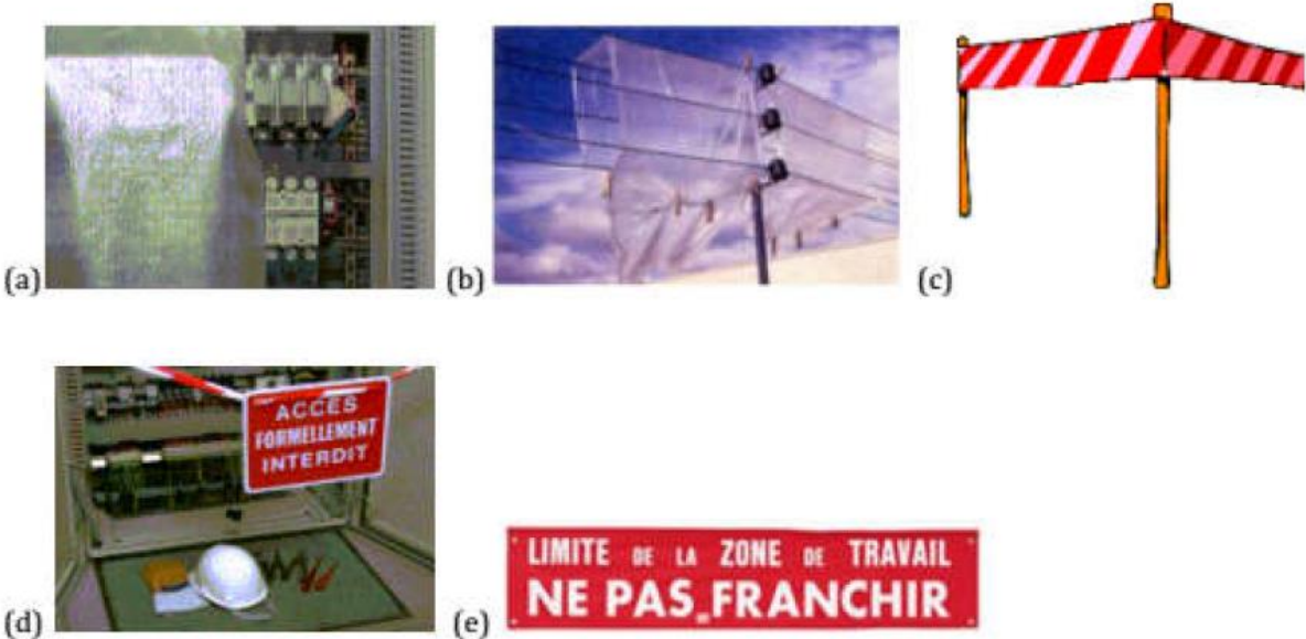
Figure III.30: temporary protection by screen (a), layers, caps and clamps (b)
