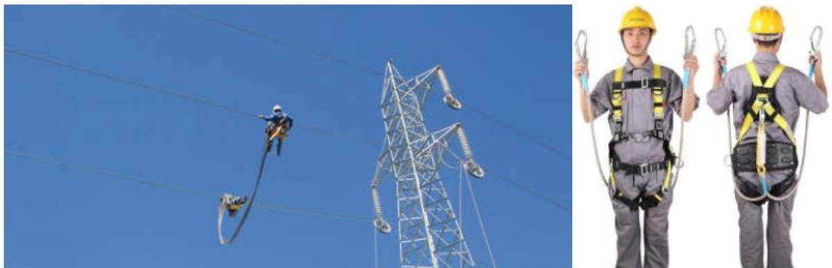
Figure III.27: Harnesses for work at height
