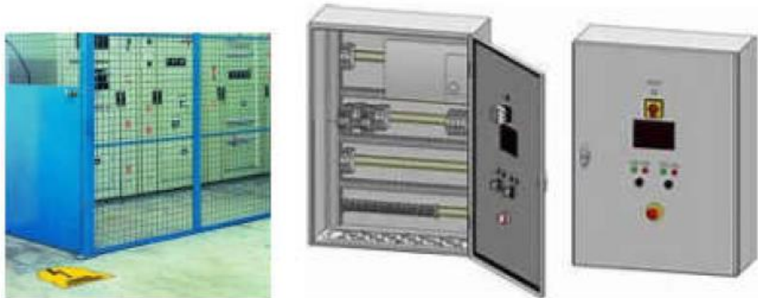
Figure III.29: Permanent protection by mesh (a) and door (b) of electrical cabinet
