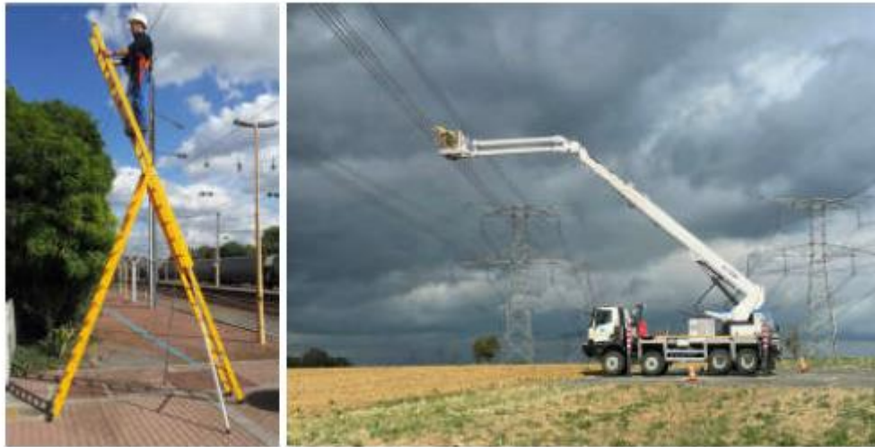
Figure III.26: Insulating ladders (a) and (b) and insulating basket (c)
