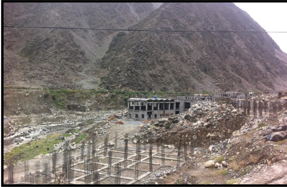
Figure I.20. Barrage de Diamer-Bhasha
