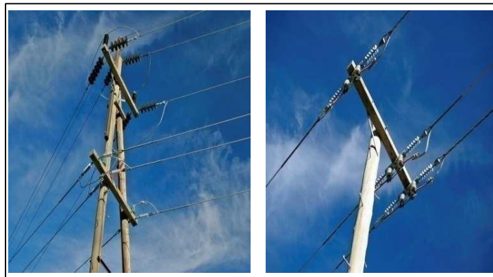
Figure I.8: Strain insulators.
