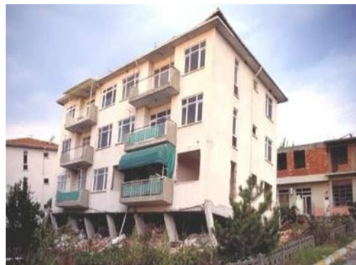
Figure I. 7: Dommages aux rez-de-chaussée souple [4]
