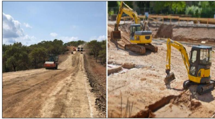
Figure 6. Examples of earthworks.
