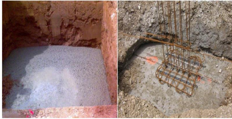
Figure 8. Clean concrete at the bottom of the foundation.
