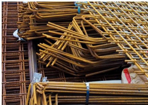
Figure 22. Reinforcement bars under construction.
