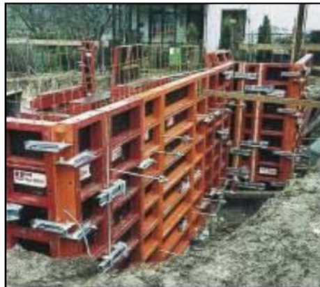
Figure 17. Public Works Scaffolding.
