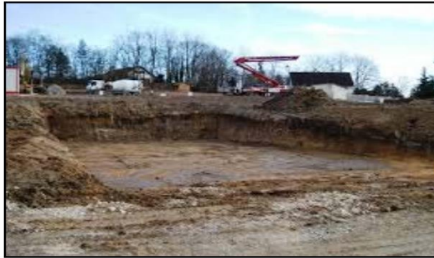
Figure 9. Full mass excavation.
