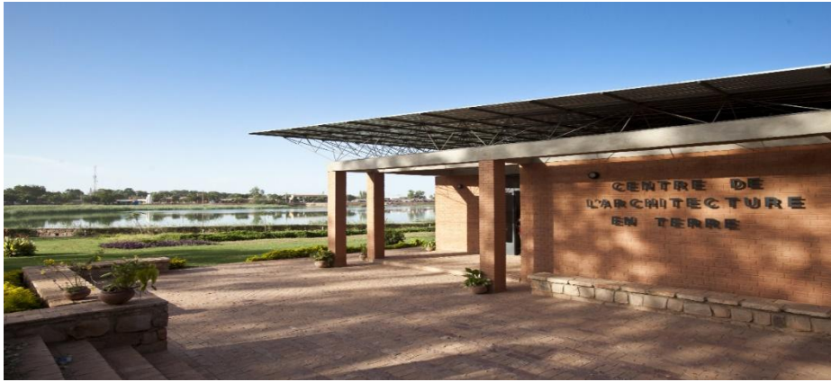
Figure I 19: The Centre for earth Architecture in Mopti, Mali
