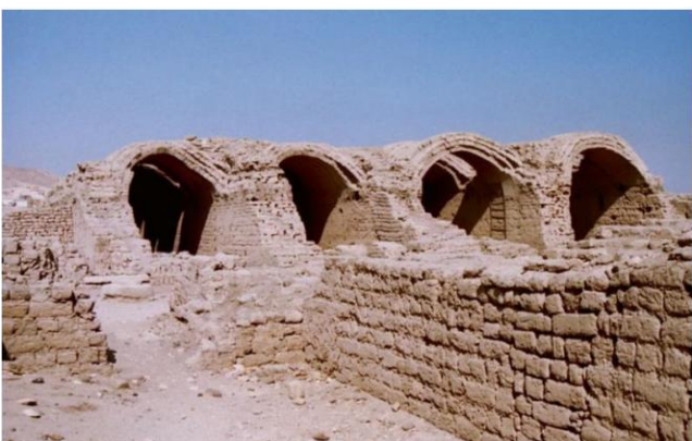
Figure I 4: Earth block vault near to Luxor, Egypt, dating to approximately 1300 BCE
