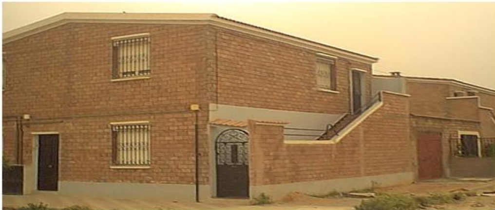
Figure I 20: R+1 semi-collective housing in Sidi Bel Abbas, Algeria [24]
