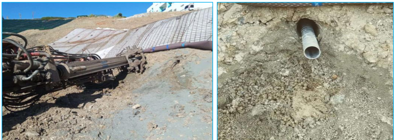
Figure I. 30 Drains Subhorizontaux
