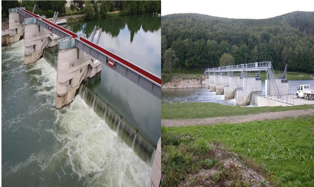
Figure I.14: Barrage mobile à clapets.
