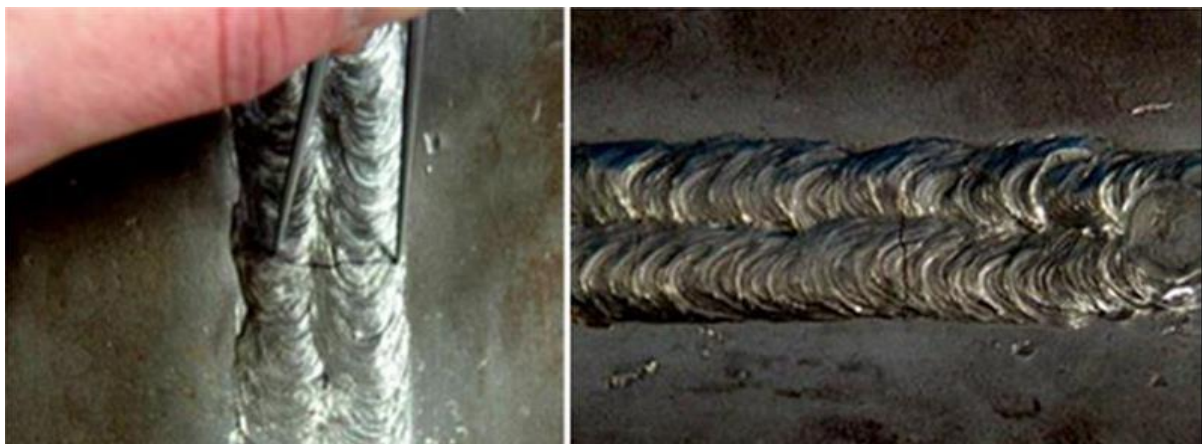
Figure. II.10 : La fissure transversale.
